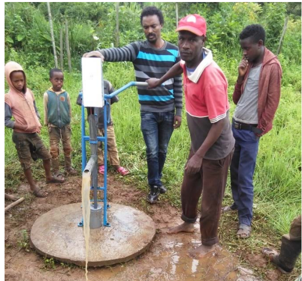
One of the 20 successful test wells installed by the project. © iDE 2019
