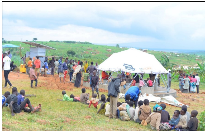
A new Hub installation near Gweke, Uganda
